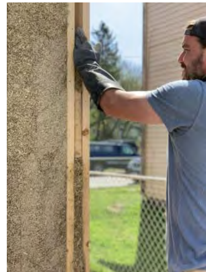
Cameron McIntosh of Americhanvre filling small cavities by hand
